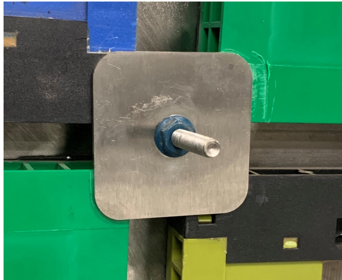
Figure 36: Tube Grid Assembly (2 1/4" SS Interior Retainer Clip)
