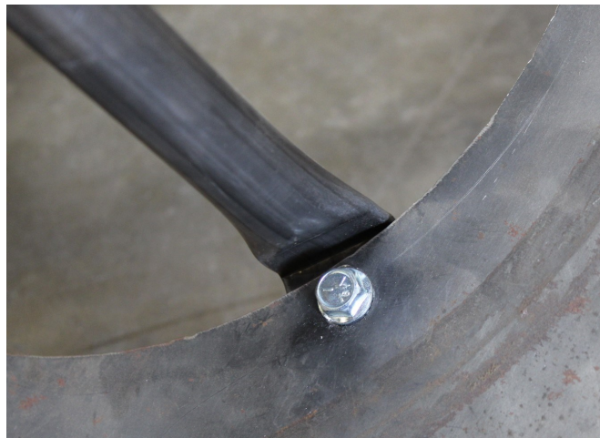
Figure 5: 5/16" Flanged Zinc Plated Mounting Bolt Assembly
