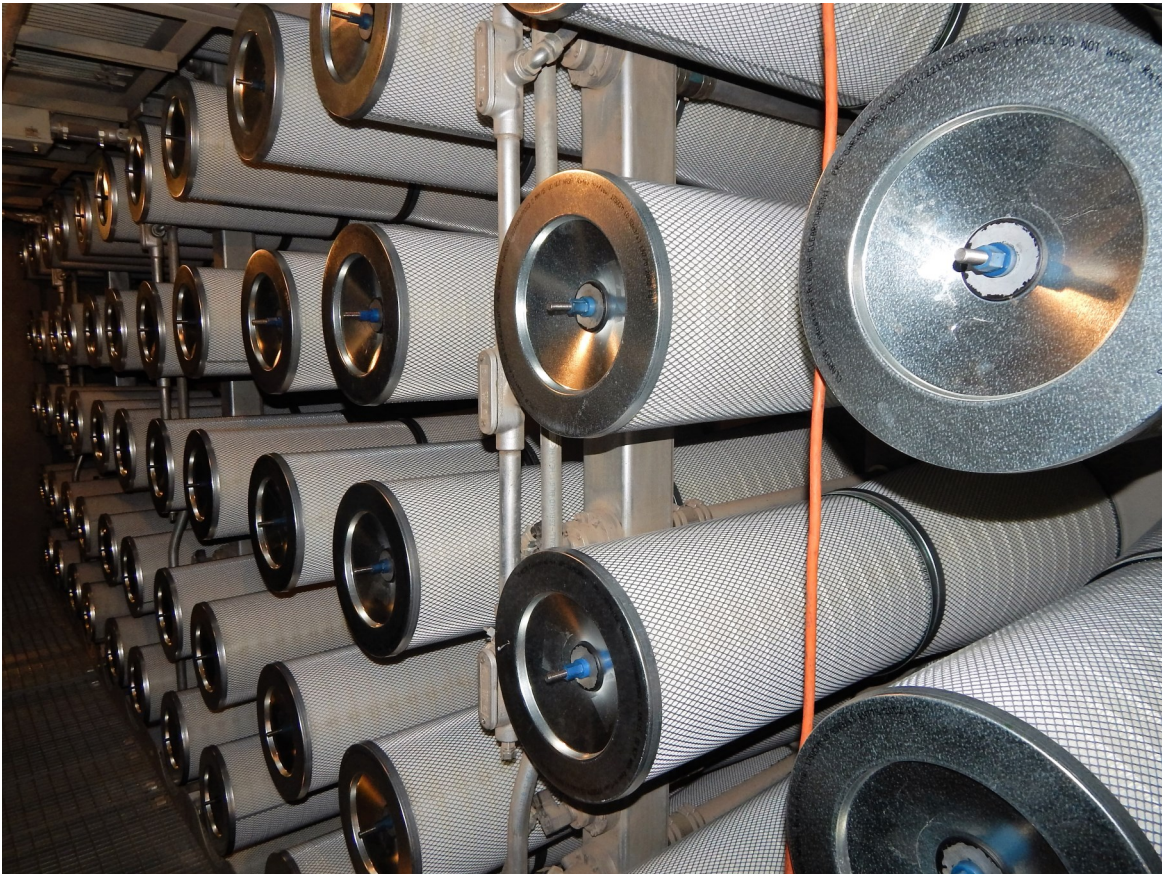
Figure 16: Installed Retainer Nuts
