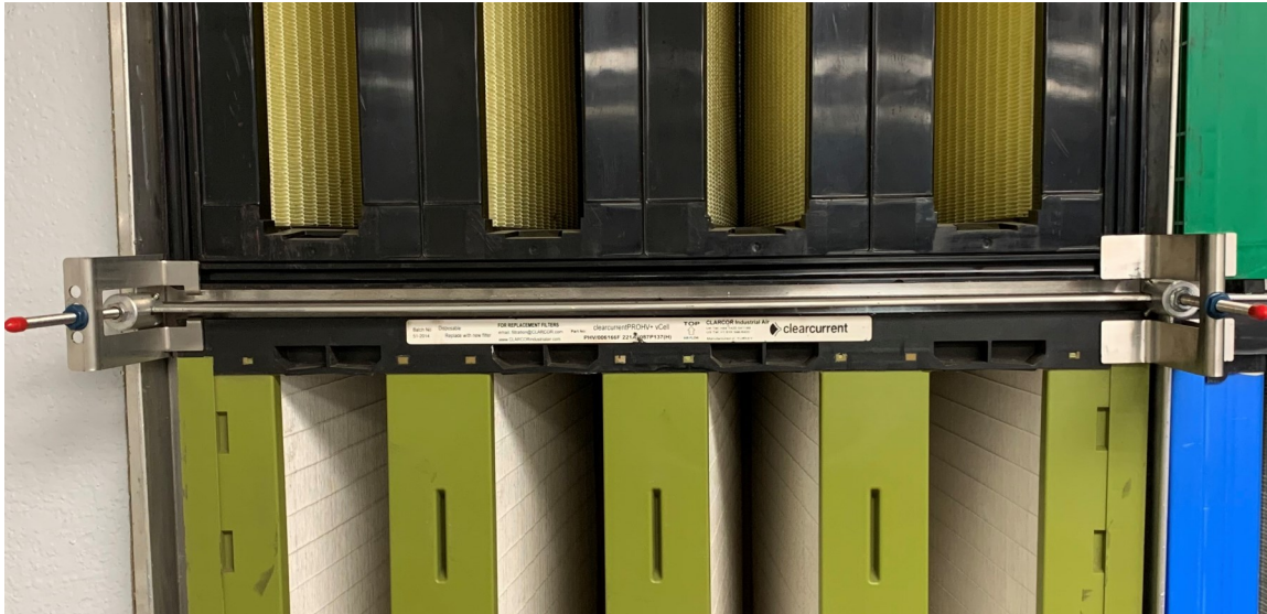
Figure 19: T-Grid Assembly
