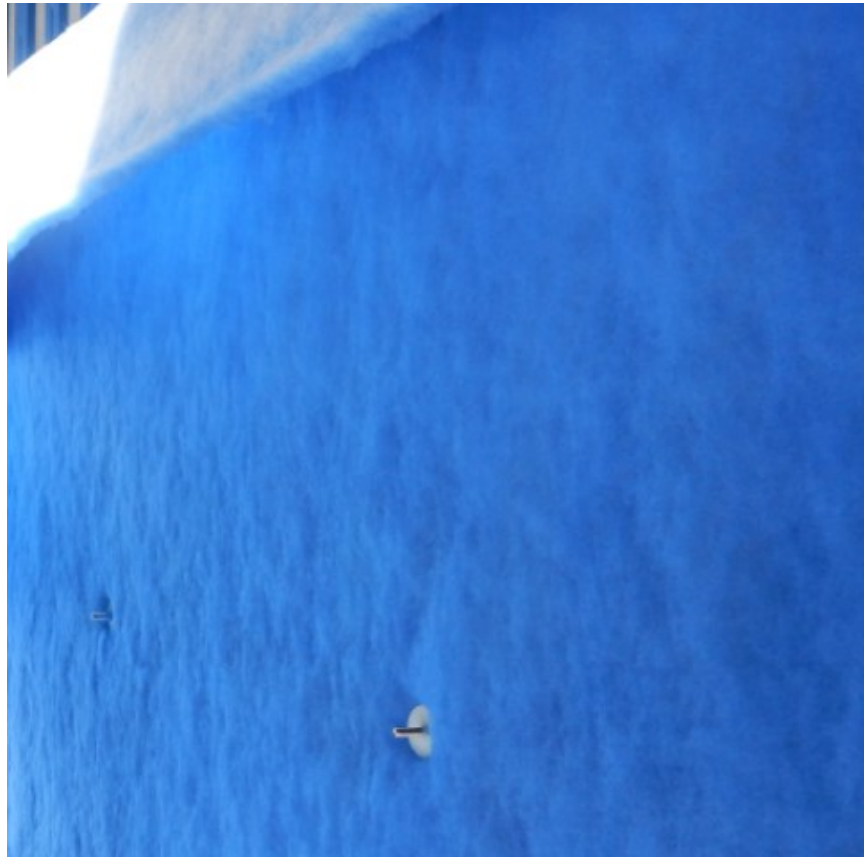
Figure 39: Coalescing Blanket Assembly
